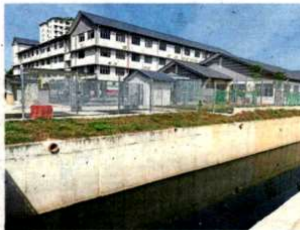
Since the monsoon drain has been upgraded, there has been no flood issues in Taman Kanagapuram.
